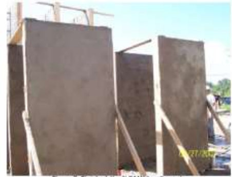
Figure 7: Finished 4' x 8' PSM50 wall panels
