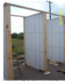
Figure 2: Finished wood frames with 4' x 8' panels ready for spray mortar application
