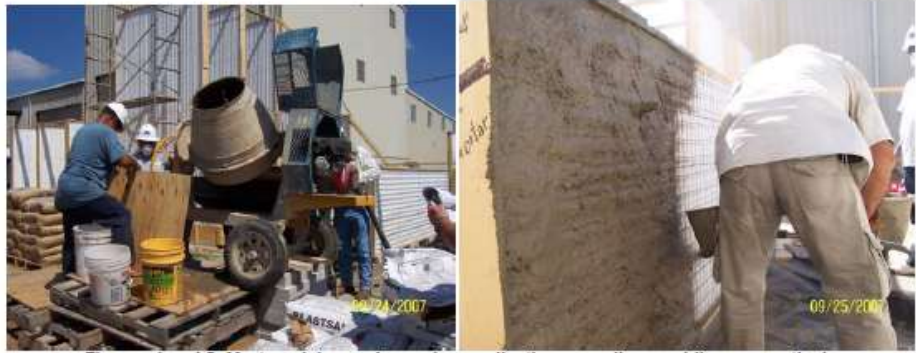
Figures 4 and 5: Mortar mixing and spraying application on wall assemblies, respectively
