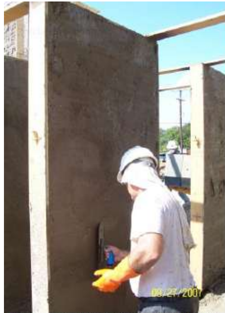
Figure 6: Smoothing out mortar after spraying
